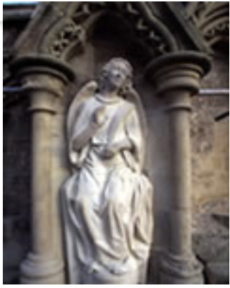
New angel on West Front carved by Jason Battle from Chicks Grove Stone, 1.60m tall.
