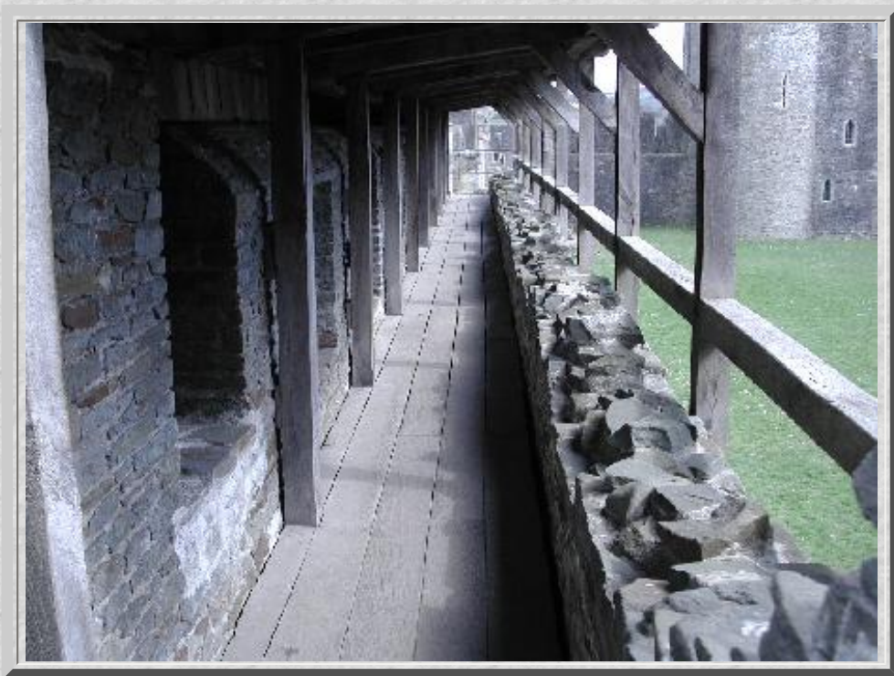
Restored parapet on the north side of the inner ward.
