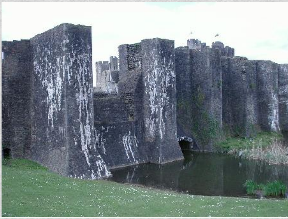
View of the three great towers along the northern dam.
