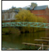
Bridge A bridge over the River Avon
