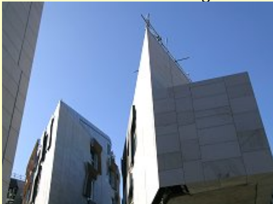
The Tower Buildings
