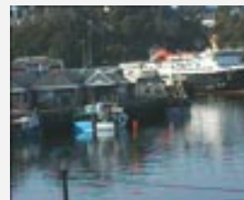
South Pier - ferry terminal
